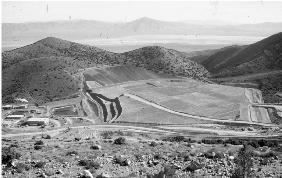
**Figure 4** Valley Fill Heap Leach - Silver Heap Leach at Rochester, Nevada. Much of the process solution is stored within the heap, behind the dam which can be seen at the downslope (left) edge of the heap.
