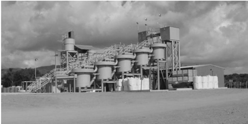
**Figure 9** Five-stage carbon adsorption column plant (CIC plant) at Glamis Gold's San Martin, Honduras project. There are two parallel column trains (one is behind the other in this view). The plant can process up to 900 cu m of solution per hour, and is sized for an operation that processes up to 20,000 tonnes of ore per day.
