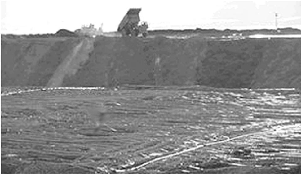
**Figure 5** Truck dumping an upper 10 meter lift of run-of-mine ore on top of a lower lift that has already been leached.
