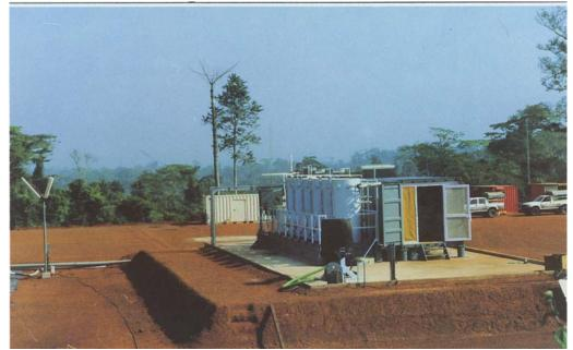
MODEL 30 CARBON ADSORPTION-DESORPTION-RECOVERY PLANT. 130 US GPM (30 CU M/HR) FOR PROCESSING 600-900 TONNES OF GOLD/SILVER ORE PER DAY.
