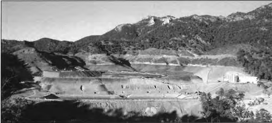
Figure 11.3-5 Valley-fill heap leach at Ocampo, Mexico
