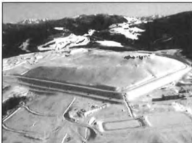
Figure 11.3-2 Heap leach installation at Brewery Creek. The open-pit mine is shown in the background. In the center of the photograph is an operating heap leach completely covered with snow.
