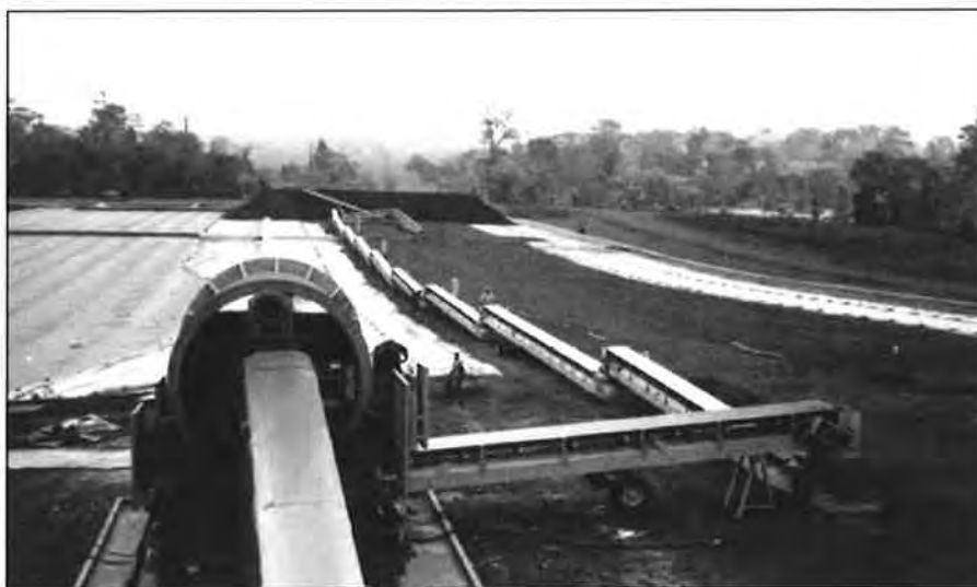
Figure 11.3-3 Agglomerating drum and conveyor stacking system with 6-m-high heap
